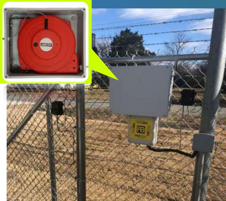
**Swing gate** – For swing gates there is no need for special equipment since the sensor cable is flexible. From the fence continue over the gate and do a U turn back to the fence. In order to bypass the gate the cable needs to be spliced with RG6 into a conduit and then spliced back on the other side. Splicing with RB-RBMCTXT Box
