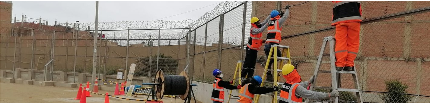
RAYSENSE INSTALLATION IN PROGRESS ON THE AIRPORT PERIMETER FENCE. CUSTOMER IDENTITY WITHHELD.
