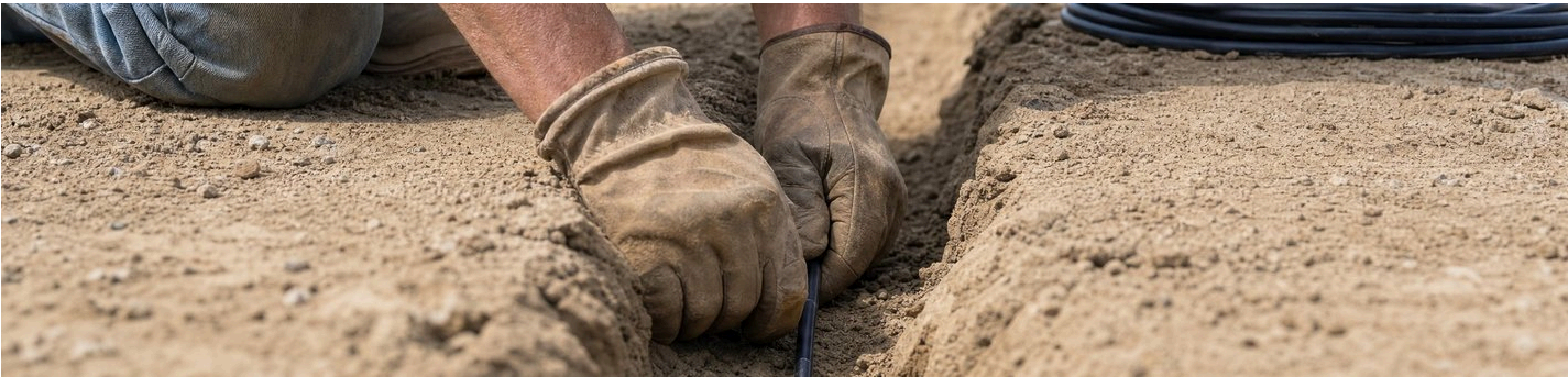
LGDS SENSOR CABLE BEING LAID IN THE TRENCH DURING BURIAL. REPRESENTATIVE INSTALLATION IMAGERY.
