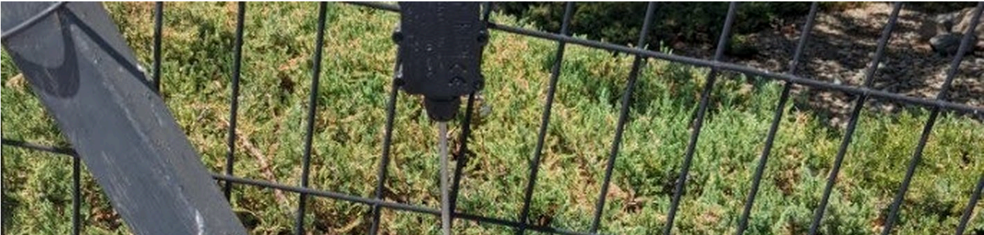
IRONCLAD SENSOR CABLE ON THE PERIMETER FENCE OF THE DISTRIBUTION SITE. CUSTOMER IDENTITY WITHHELD.
