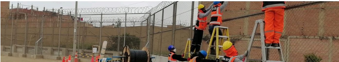
RAYSENSE INSTALLATION ON A PERIMETER FENCE. REPRESENTATIVE PHOTOGRAPHY; CUSTOMER IDENTITY WITHHELD.
