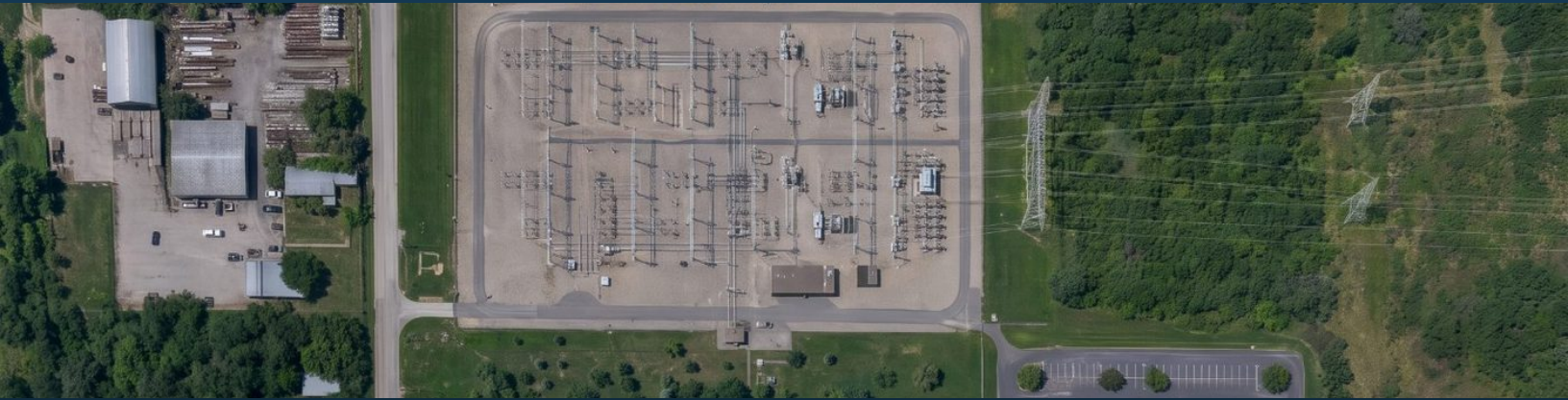
AERIAL VIEW OF AN UNMANNED TRANSMISSION SUBSTATION. ILLUSTRATIVE IMAGERY; CUSTOMER IDENTITY WITHHELD.
